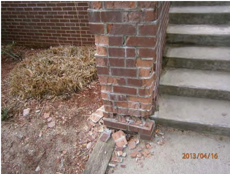
5. Bick column damage
