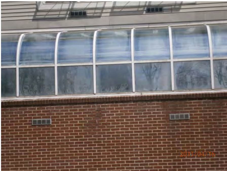
7. Atrium windows - insulated glass failure
