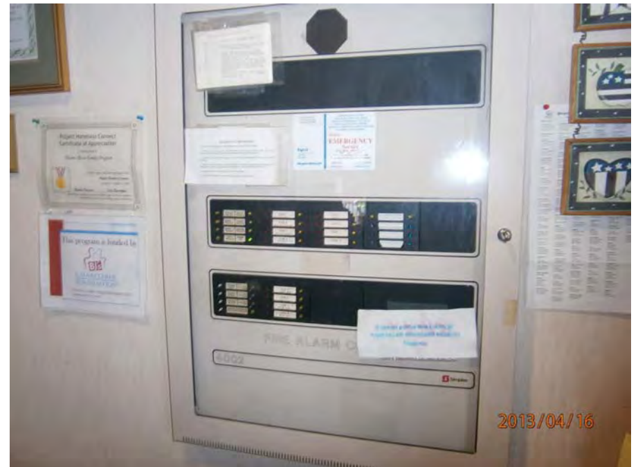
20. Zoned fire control panel
