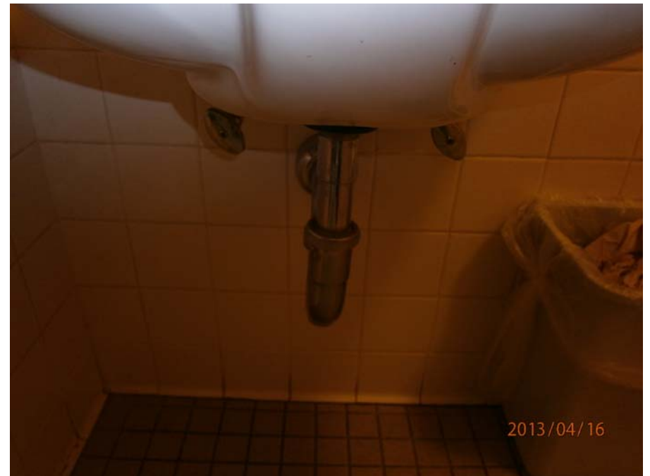
16. Accessibility - sink trap protection missing
