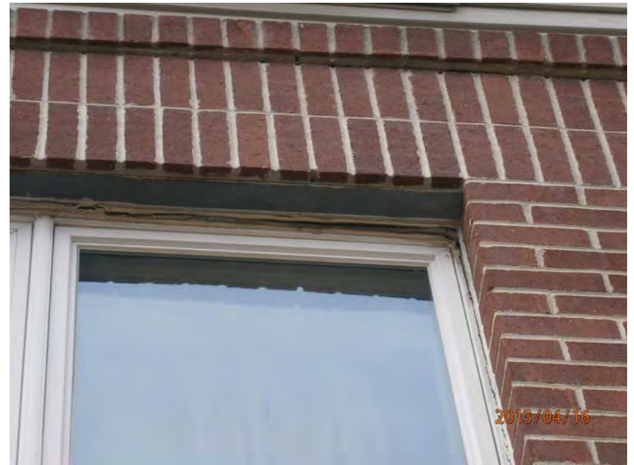
6. Window failure at lintel
