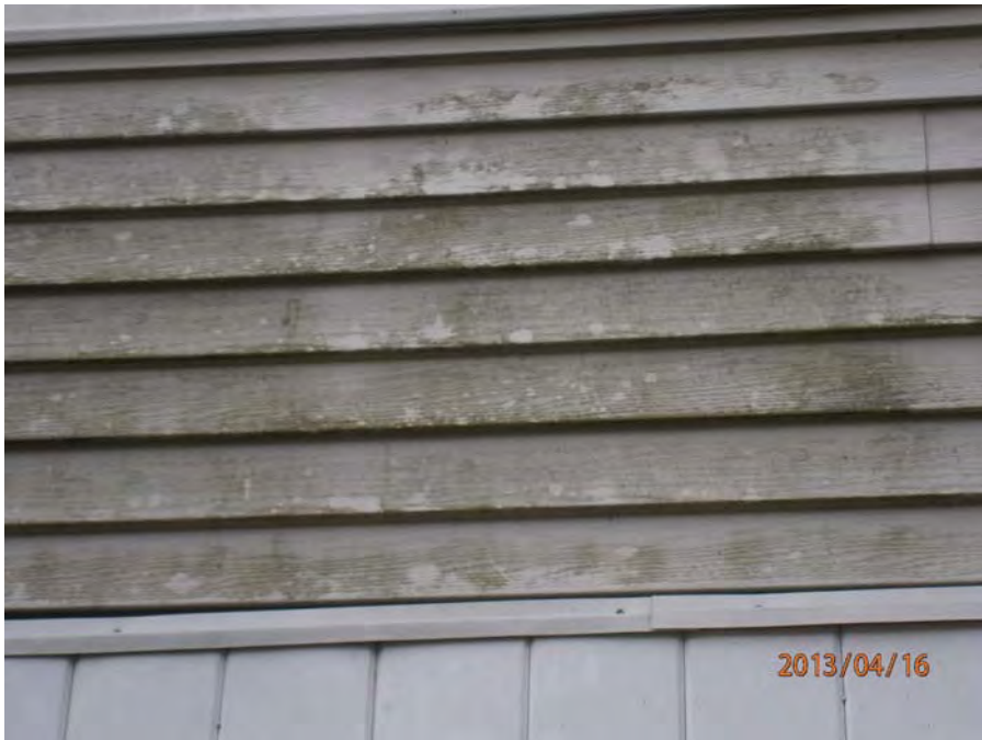
9. Vinyl siding - pressure washing needed
